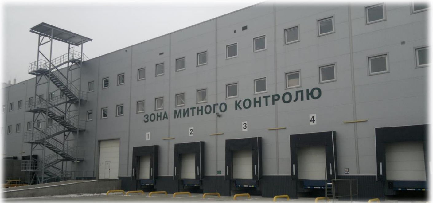
LOGISTICS COMPLEX «Inrise Logistics», Odesa region Volume of delivered products - 14 150 m 2
